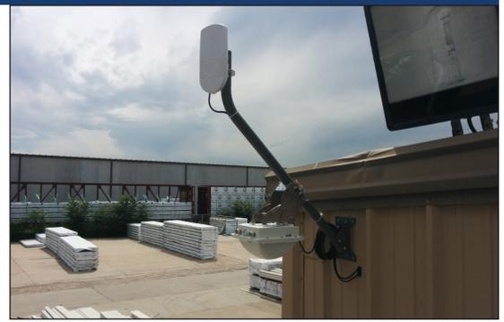
ePMP module and WLAN Access Point
